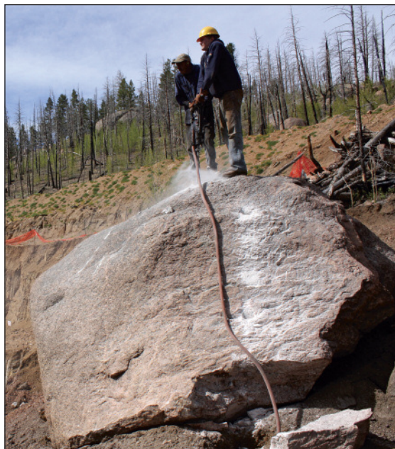
Drilling and blasting hard parts of the granite is sometimes necessary. P5M photo.
